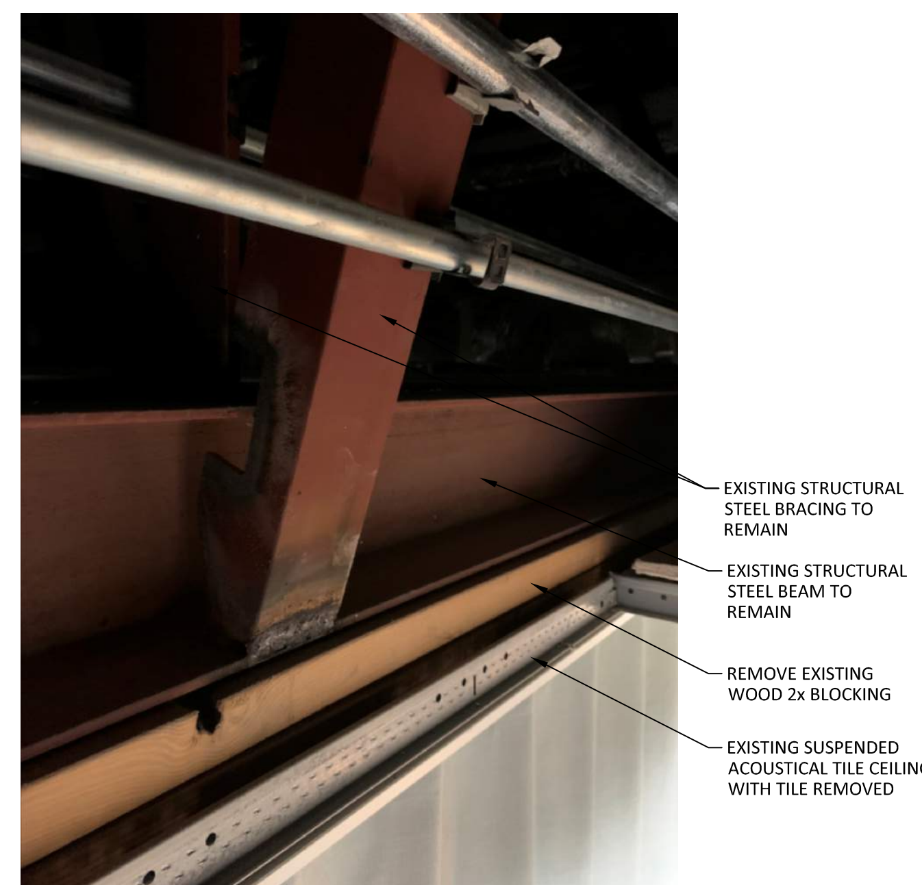
4 PHOTO ABOVE CEILING AND ABOVE THE EXISTING RETRACTABLE PARTITION WALL NOT-TO-SCALE
