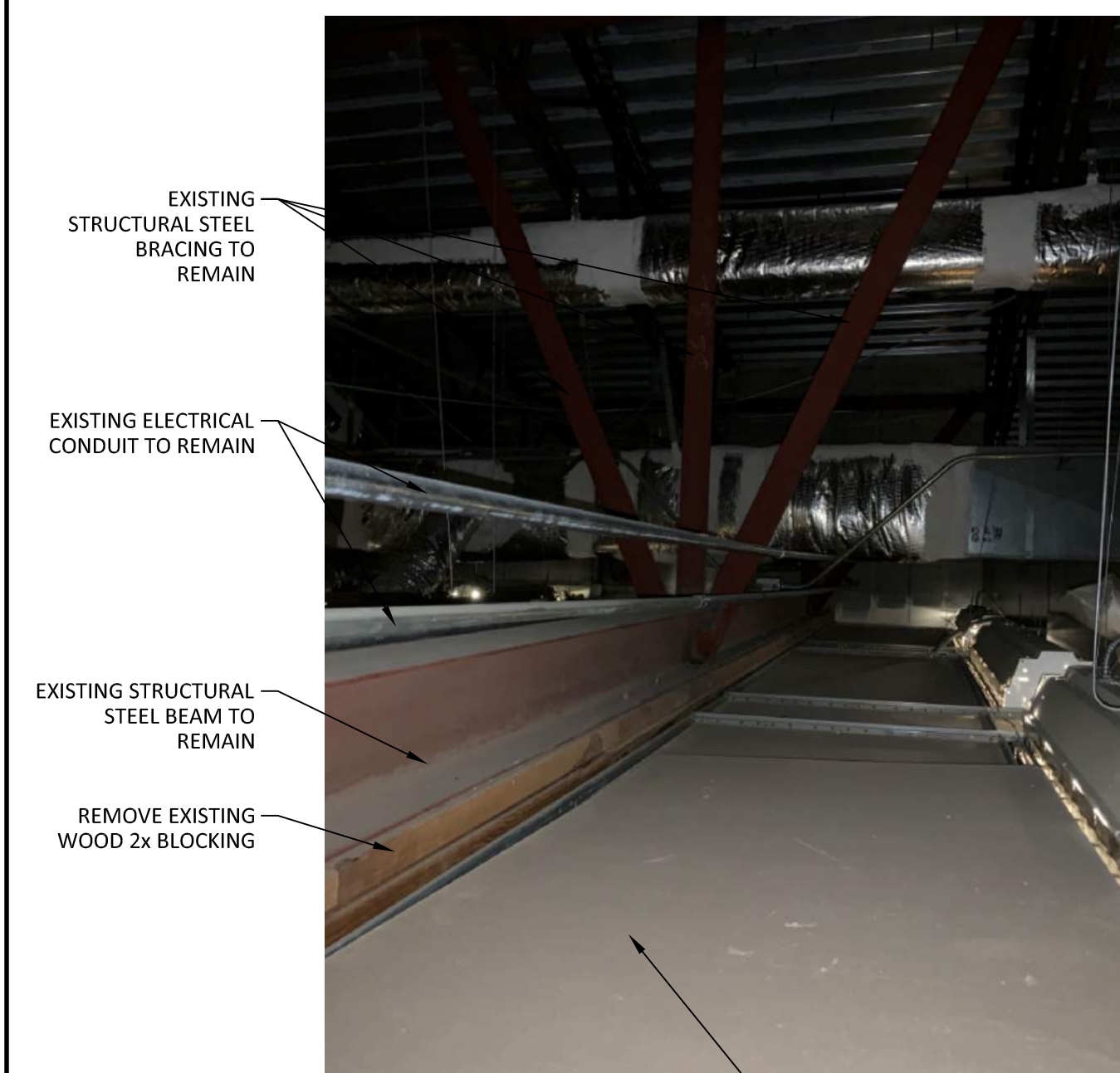
3 PHOTO ABOVE CEILING AND ABOVE THE EXISTING RETRACTABLE PARTITION WALL NOT-TO-SCALE
