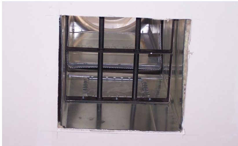
Figure 3-13 Bars on Penetration
