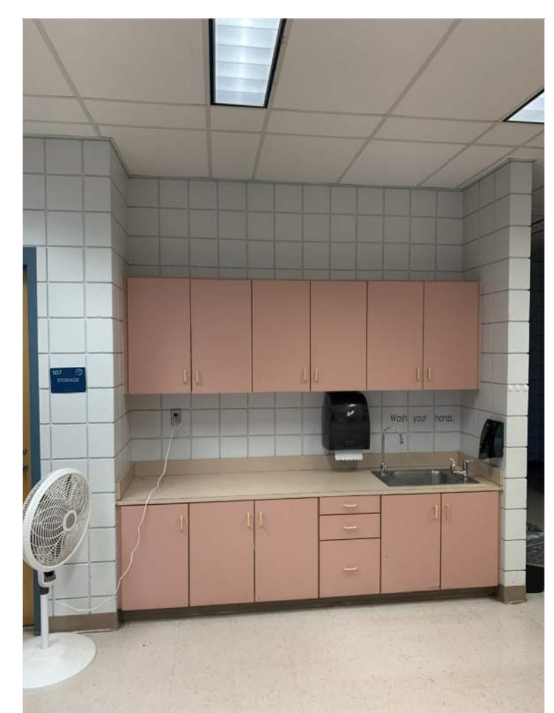
12 CLASSROOM MILLWORK - TYPE-2 EXAMPLE EXISTING CONDITIONS
