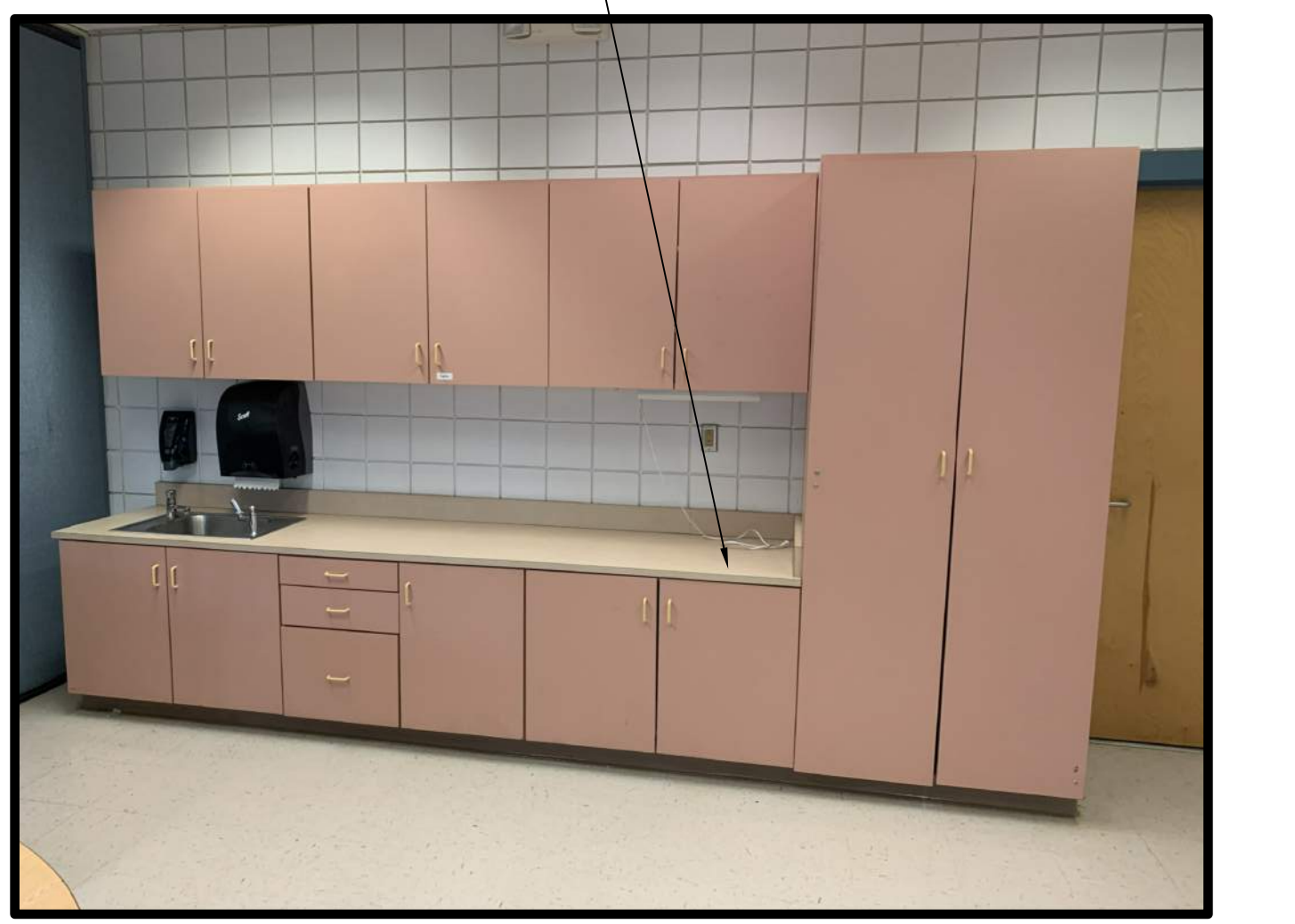
10 SPECIALTY CLASSROOMS - MILLWORK
