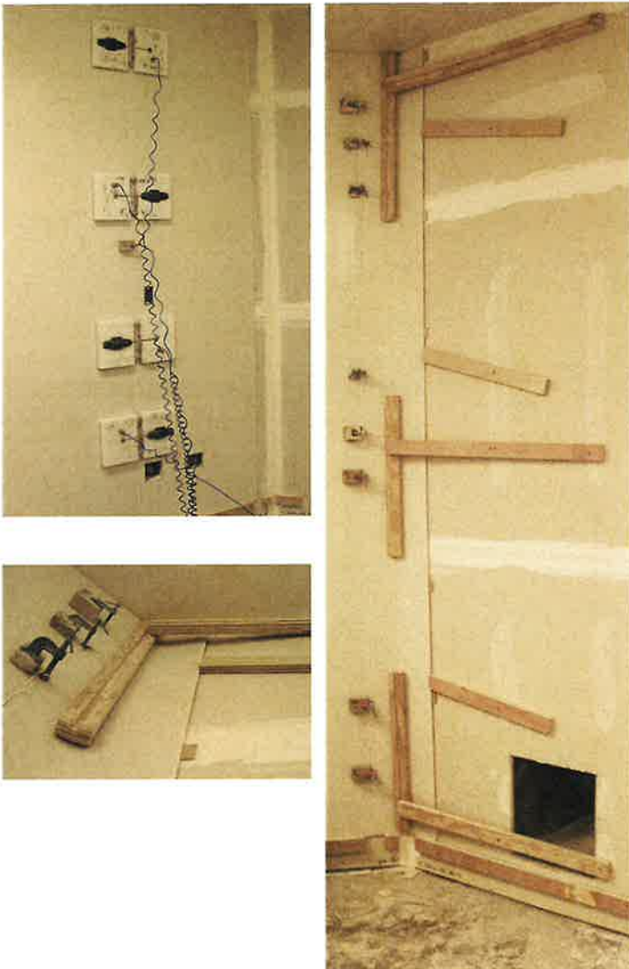
FIGURE P-1: CLAMPING SEAMS
