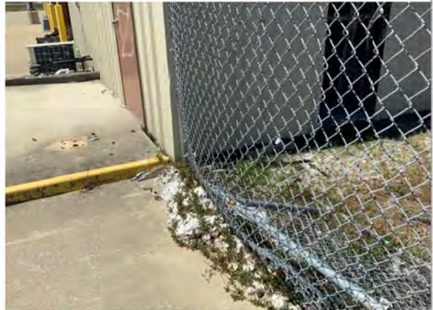
Soil Boring Location #2
