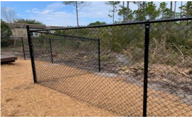
Panic Gate – Black Powder Coated Panic Gate with self-closing hardware and Dtek panic bar (Industrial Grade)
